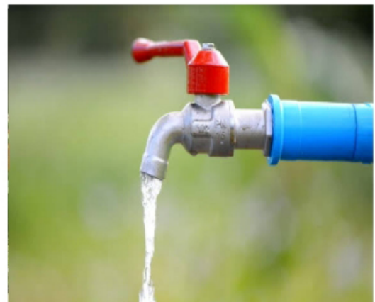
Water flowing through pipe
